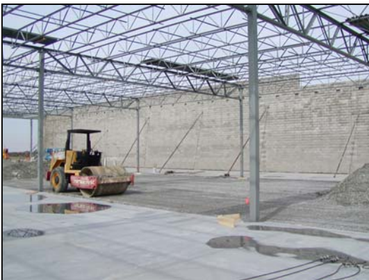
Fig. 7 View from Inside Target Store
