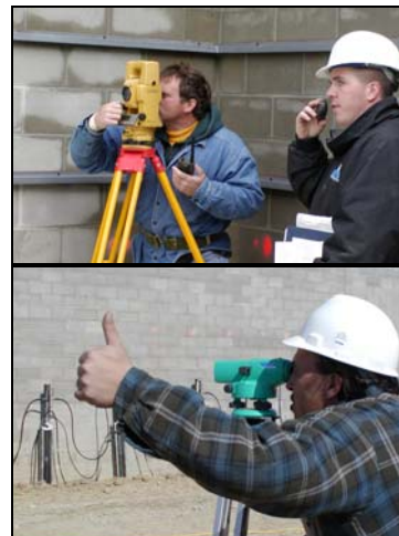
Fig. 13 Monitoring Wall Movement During Lifting Phase
