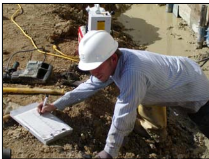
Fig. 12 Logging Pier Depth and Hydraulic Pressure
