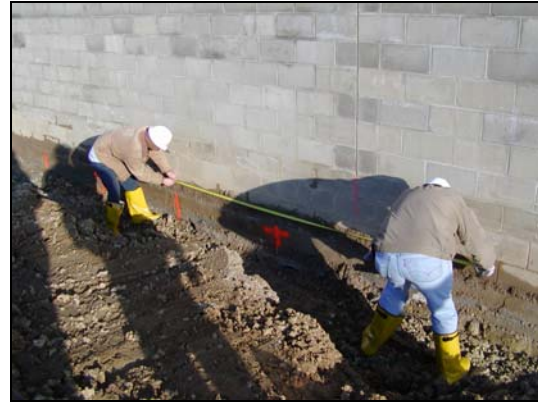
Fig. 9 Marking Bracket Positions Along Foundation Walls
