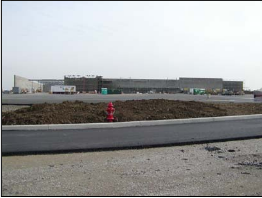
Fig. 6 Distant View of Target Store Site
